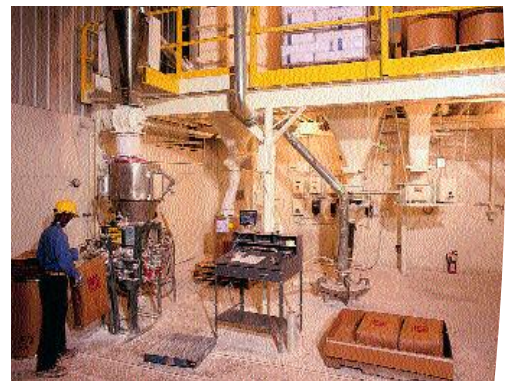
Micro-Jet work station with valve bag packaging. Each work station is designed for maximum flexibility in milling and packaging equipment.
